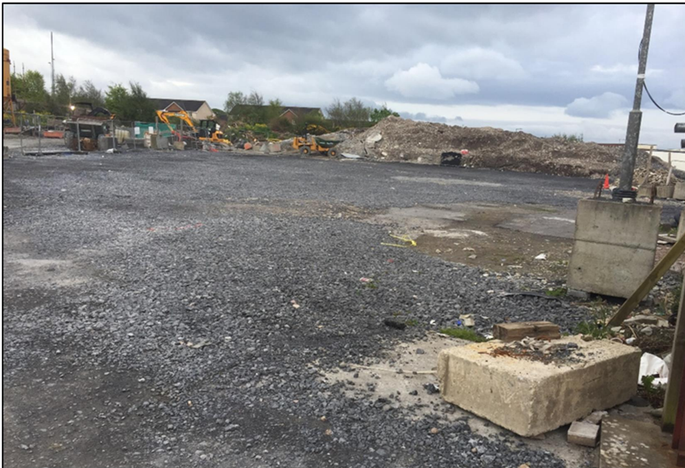
Plate 3.2: Spoil and Bare Ground (ED2)
